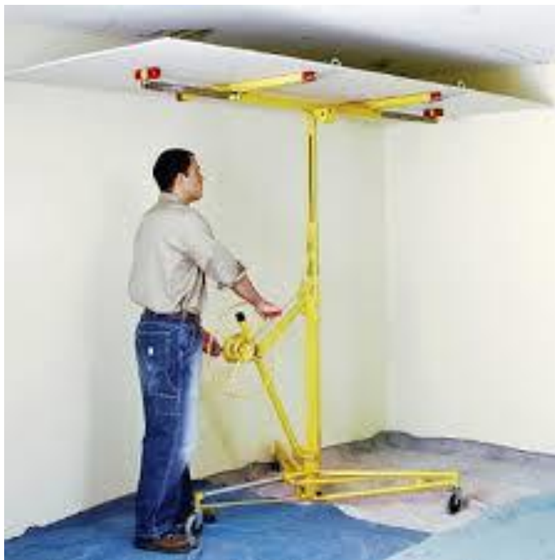
Figure 9. Example of a drywall lift. Adapted from “How to Hang Drywall on Ceiling with a Lift,” by Baixar Musica, n.d. Copyright 2015 by Baixar Musica.
