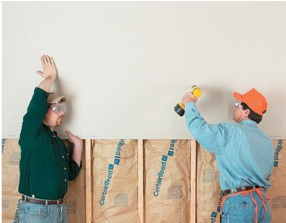
Figure 5. Workers attaching drywall to framing.
