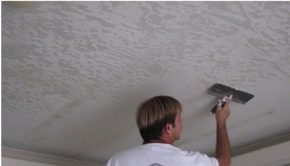
Figure 7. Worker applying drywall texture. Adapted from “Skip-Trowel Texture,” by K. B. Marks, n.d. Copyright n.d., by Bill Marks Painting.
